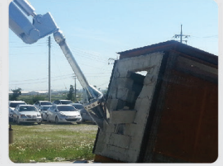
Demolition of Concrete wall
