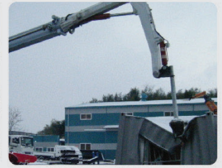
Demolition of Container
